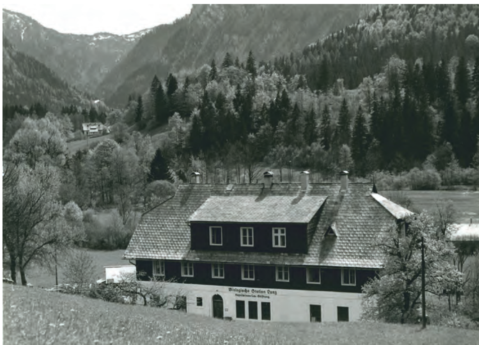
Fig. 93: Biological Station in Lunz
